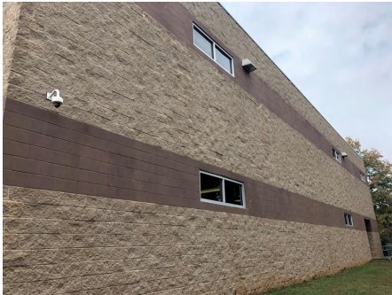
7). Exterior Elevation - Jan 25, 2020
