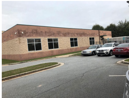
5). Exterior Elevation - Jan 25, 2020
