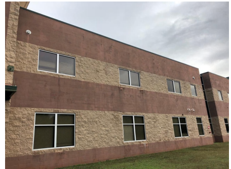
6). Exterior Elevation - Jan 25, 2020
