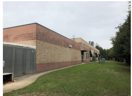
9). Exterior Elevation - Jan 25, 2020
