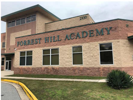
10). Exterior Elevation - Jan 25, 2020
