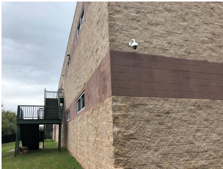
4). Exterior Elevation - Jan 25, 2020
