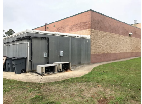
3). Exterior Elevation - Jan 25, 2020
