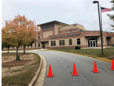
2). Exterior Elevation - Jan 25, 2020
