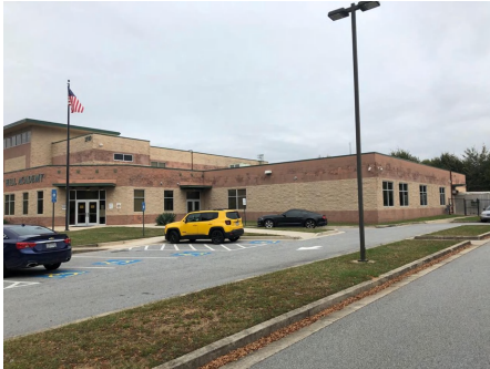
1). Exterior Elevation - Jan 25, 2020
